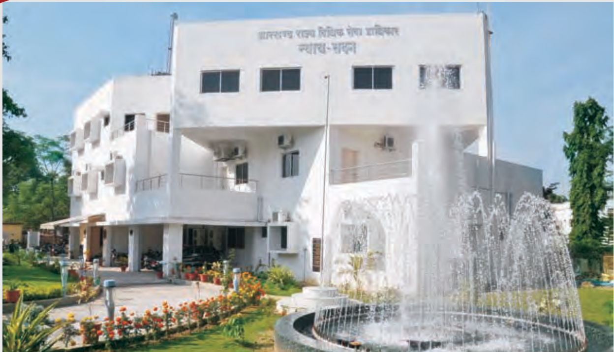
"Nyaya Sadan", present building of Jharkhand State Legal Services Authority
