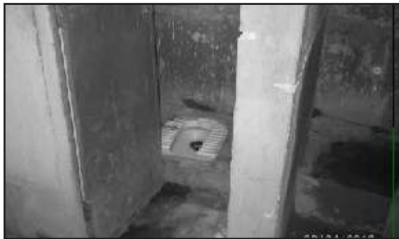
Inadequate & unhygienic condition of the toilet block on Ground Floor of KGBV School, Bharno
