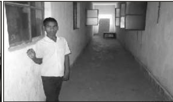
The new building with plaster peeling off from the floors, the building in an unusable condition, the toilet block without any water and with jammed pipes.
