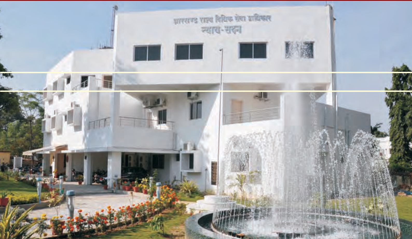
PRESENT JHALSA BUILDING
